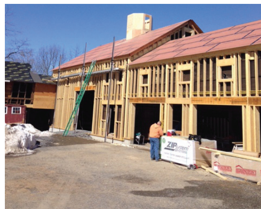
Above: A protective exterior “shell” was built over the existing barn’s siding. Left: Folding metal doors, replete with large windows, is the main entryway into the barn. Also depicted in this photo is the finished cupola.
